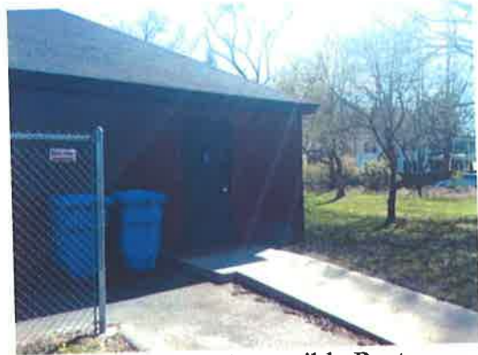
Handicap Accessible Restroom
